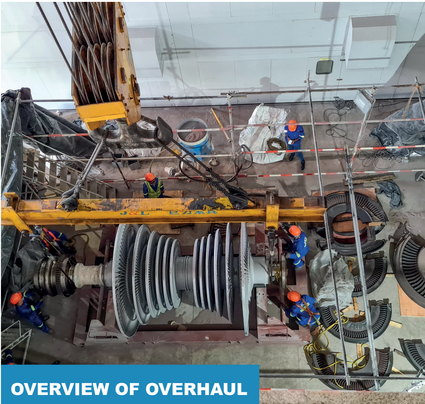
Turbine Repairs
