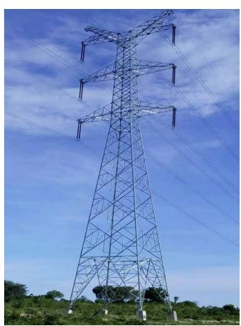
SZA2 Tower after erection and accessories installation
