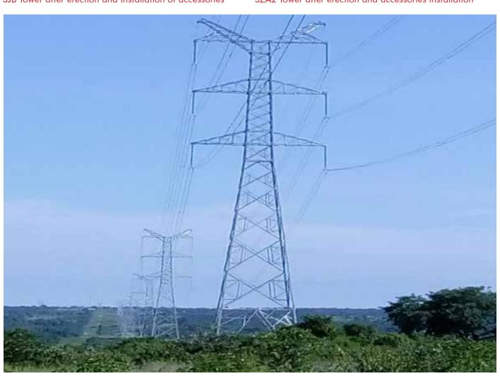
After conductor pulling and accessories installation between Towers G107-G94
