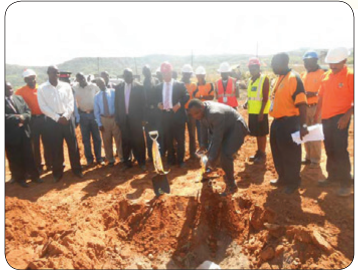
Sinazongwe Member of Parliament Honourable Richwell Siamunene also lays ground at the TPP construction site on 12th May 2012
